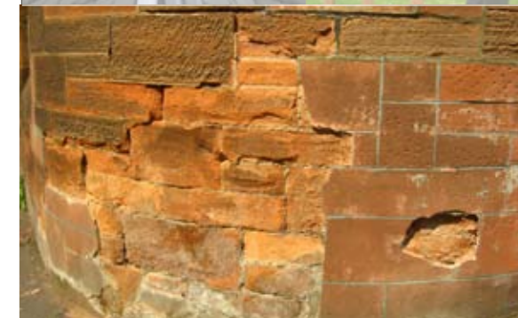
Stone decay accelerated by cement at Brechin's Bar
